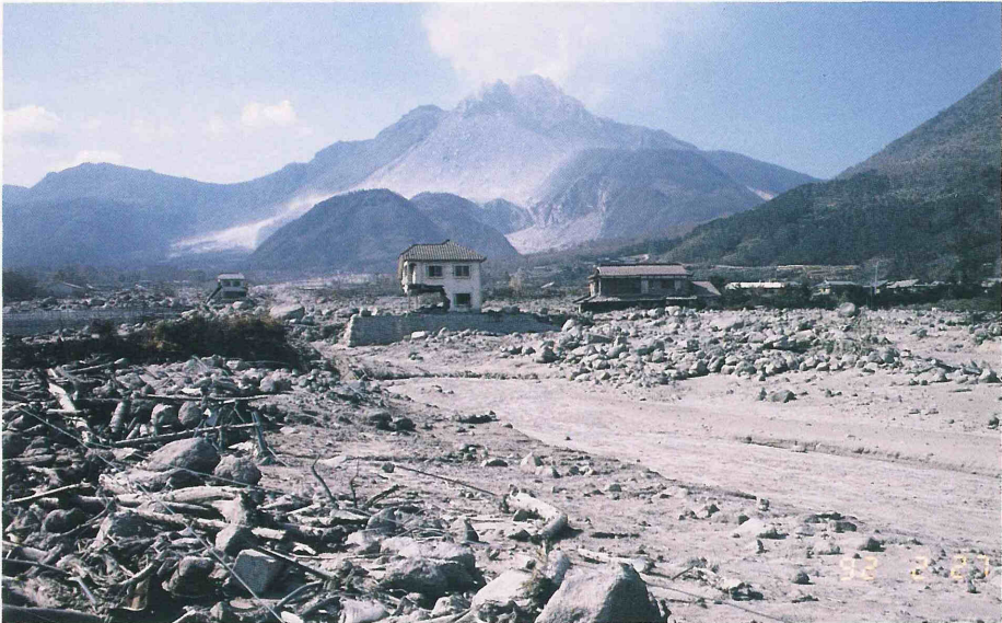
Fig. 11-2. Broken houses by the debris flow on 30 June. Houses have been still left broken in the limited-entry zone. (by Hirano, 22 February 1991).
