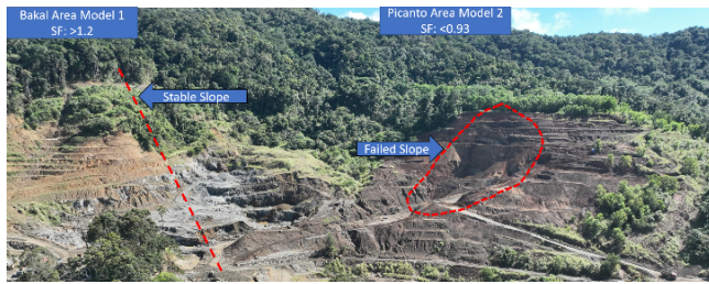
Figure 5. Photographs of a stable slope (left side) and a failed slope (right side) in the study area.
