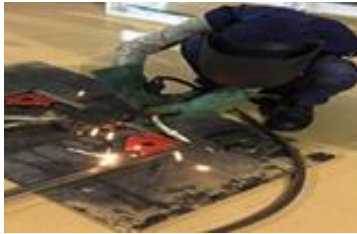
Fig. 10. Attach framework used for Metal Inert Gases (MIG) welding.
