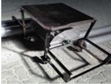
Fig. 11. Finishing process by painting the framework to avoid corrosion.
