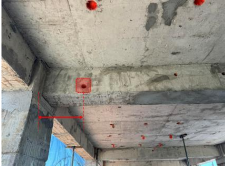
Fig. 2. Typical beam penetration detail.
