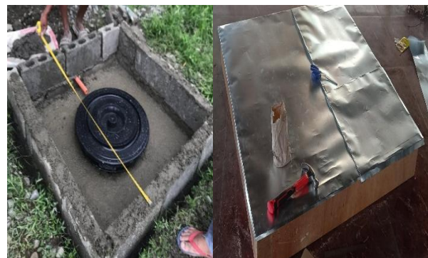
Figure 6. Surface enclosure & vault door frame
