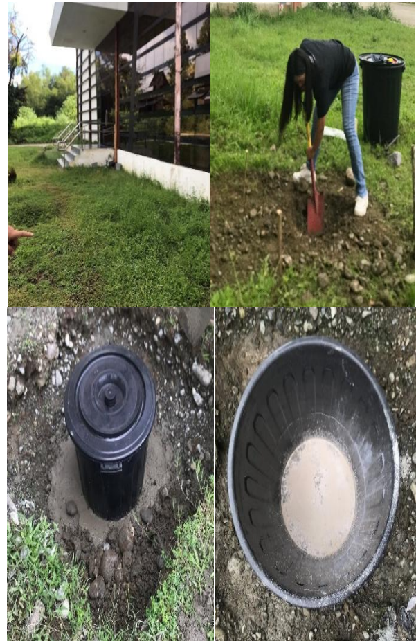
Figure 4. Site selection & vault hole excavation
