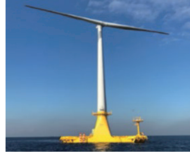
Fig. 11 Floating wind turbine “Hibiki” 2)
