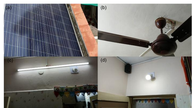
Fig. 3: Installation at small house (a) single solar panel; (b) and (c) DC ceiling fan; (c) LED tube light and (d) Battery
