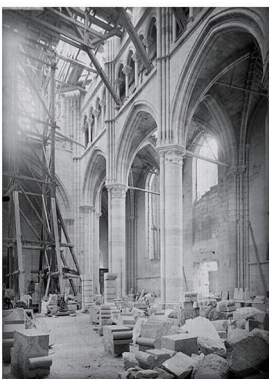
Fig. 9. Case No. 15. Soissons Cathedral, photograph showing the work after 1918
