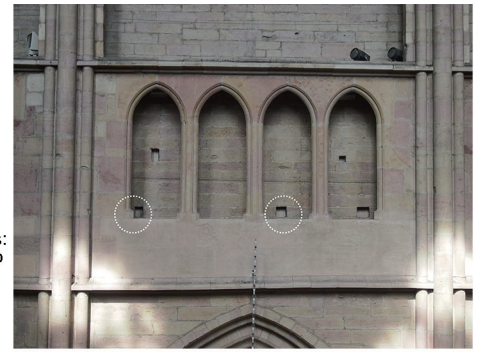
Fig. 18. Dijon, abbey church of Saint-Bénigne. Left: Plan with indications of putlog holes Right: Triforium with indications of putlog holes
