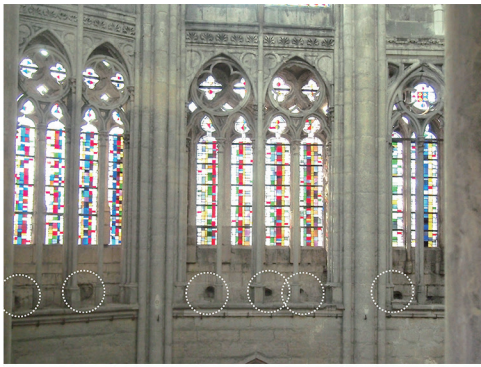
Fig. 17. Beauvais Cathedral, choir. Triforium with indications of putlog holes
