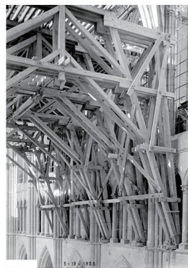
Fig. 10. Case No. 16. Reims Cathedral, photograph showing the scaffolding in 1922
