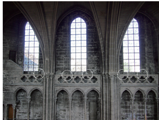
Fig. 20. Chalon-sur-Saône Cathedral. Choir, clerestory and triforium with indications of putlog holes
