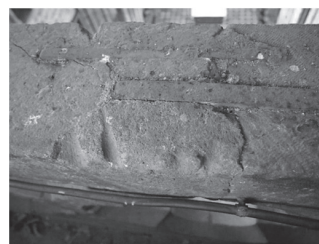
Fig.7 Chalon-sur-Saône Cathedral, choir, balustrade of the clerestory passage. Traces of cords.
