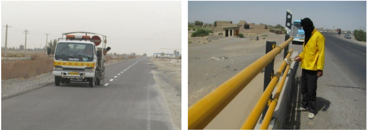
Figure. 2.7. Remarking Road surface and repairing bridge fences after dust storm (Miri & Middleton. 2022).
