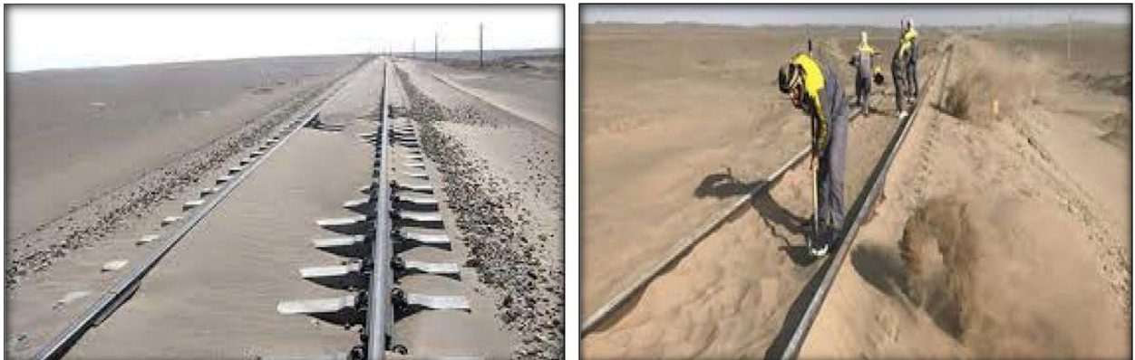
Figure. 2.8. Sand deposition on the rails and cleaning (Miri & Middleton. 2022).
