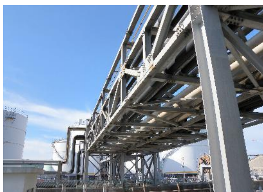
Fig. 1-1 The hot-dip coating used in the trestle bridge.
