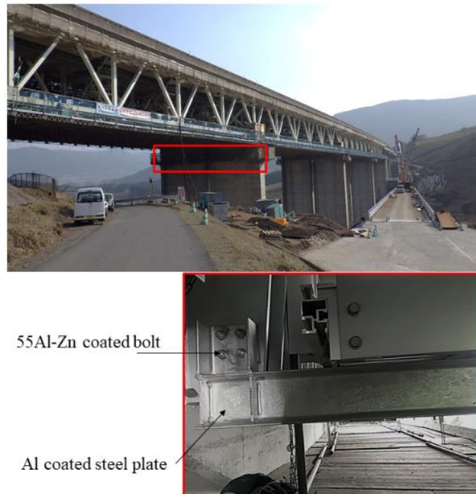
Fig. 4-1 Inspection device for maintain management of bridge substructure.
