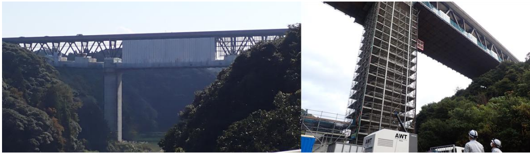
Field photograph of the bridge where AWT processing will be directly applied.
