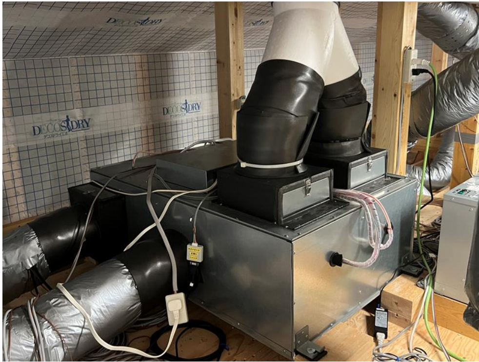
(c) ERV's photograph after installation
