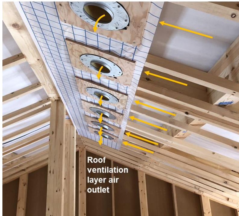
(c) Roof ventilation layer outlet
