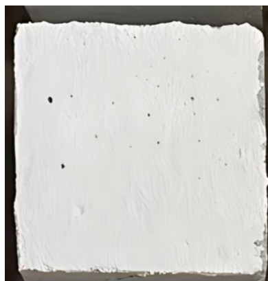
Fig. 8. Commercially available \text{Mg}(\text{OH})_2 coating on concrete specimen
