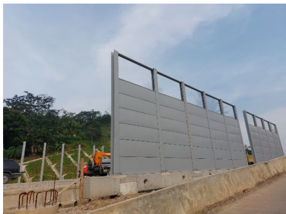
Fig. 2: Composite noise-reduction structure made from metal plate and concrete for Jakarta-Bandung high-speed railway project, Indonesia.
