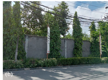
Fig. 1: Noise-reduction structures made from concrete: (a) concrete, brick, and river stone; (b) concrete and brick.
