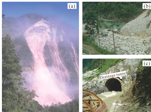
Figure 14. (a) Full view of Baishi landslide when sliding on July 30, 2007; (b) landslide dam and barrier lake; (c) drainage tunnel releasing the water of barrier lake.
