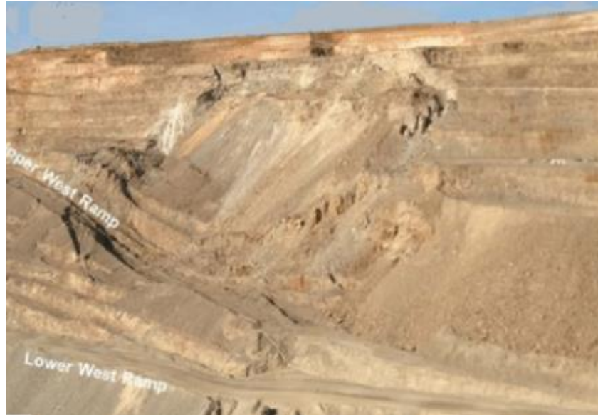
Figure 1. 23 Surface subsidence caused by sub-level cave (SLC)
