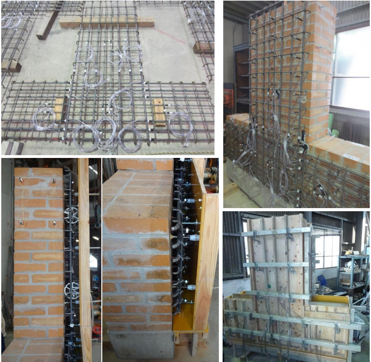
Figure 7.4: Laying of reinforcement and casting of RC wall process
