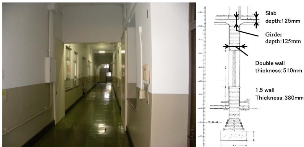
a) Inner wall of existing structure
