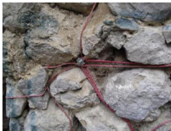
Figure 2.23: Application of reticulatus system on stone masonry adopted from (Borri et al., 2011)
