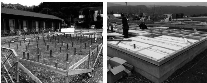
Photo 1 Timber pile foundation (Left) and reinforced concrete foundation in Kumamoto (Right) of temporary housings 仮設住宅 従来の木杭基礎(左)と熊本のコンクリート基礎(右) 注 1)
