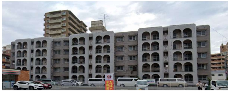
Figure 5. 1 Rear view of Hikari Building
