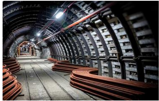
d. Steel arches
