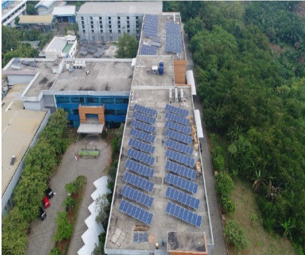
Fig. 2: View of 93.6 kWp rooftop PV system at Building 625, Puspipstek, Serpong, South Tangerang
