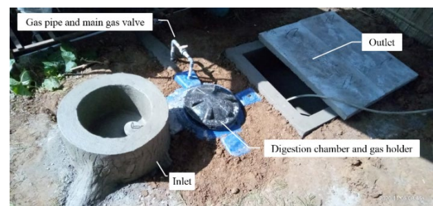
Fig. 3: Completed construction of small-scale low-pressure biodigester.
