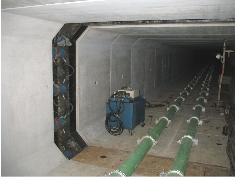
Fig. 14 Rectangular intermediate jacking station.
