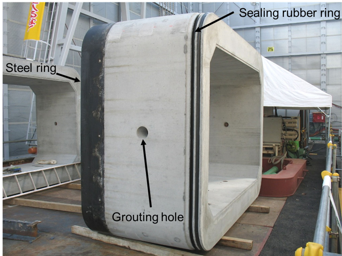
(c) Box culvert
