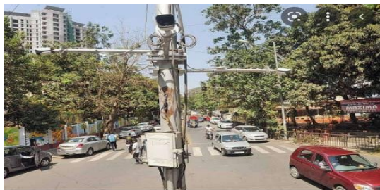
Fig. 18: Improper position for density counting camera.
