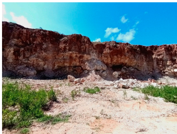
Figure 6. Near-vertical slopes from excavation.
