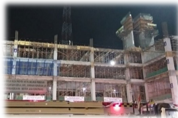
Construction phase of building
