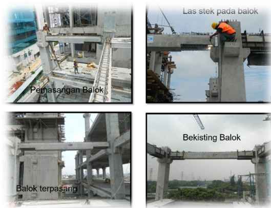
Construction phase of building
