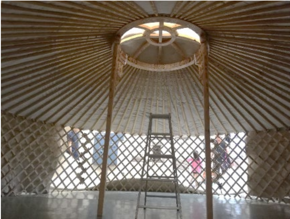
Fig. 3.3 Assembled wooden structure covered by a felt sheet
