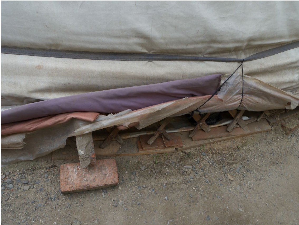
Fig. 2.14 Photo of the roll-up hem of ger envelope
