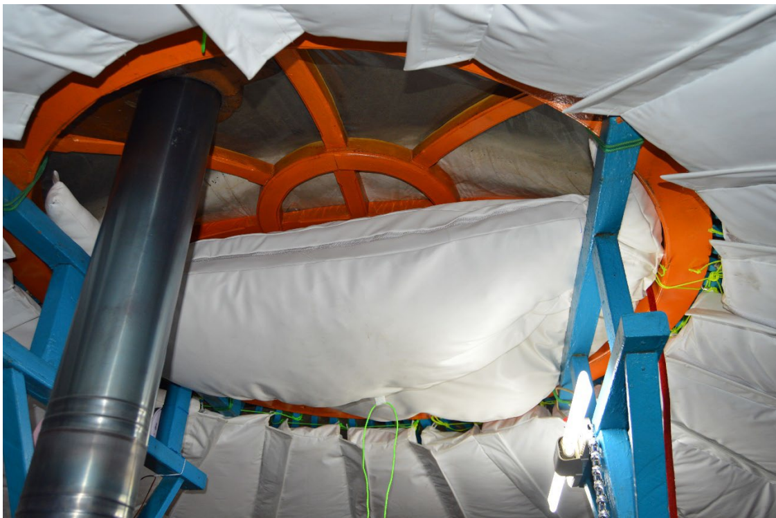
Fig. 3.21 Insulation for the skylight /toono
