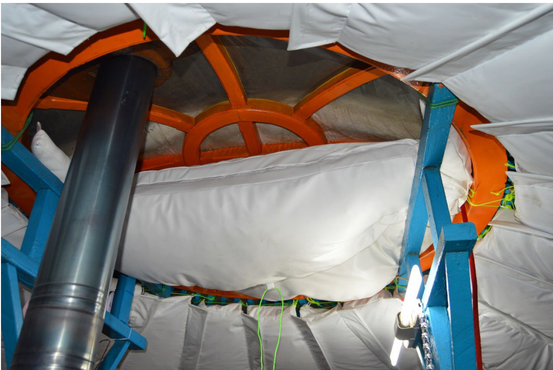
Fig. 3.21 Insulation for the skylight /toono
