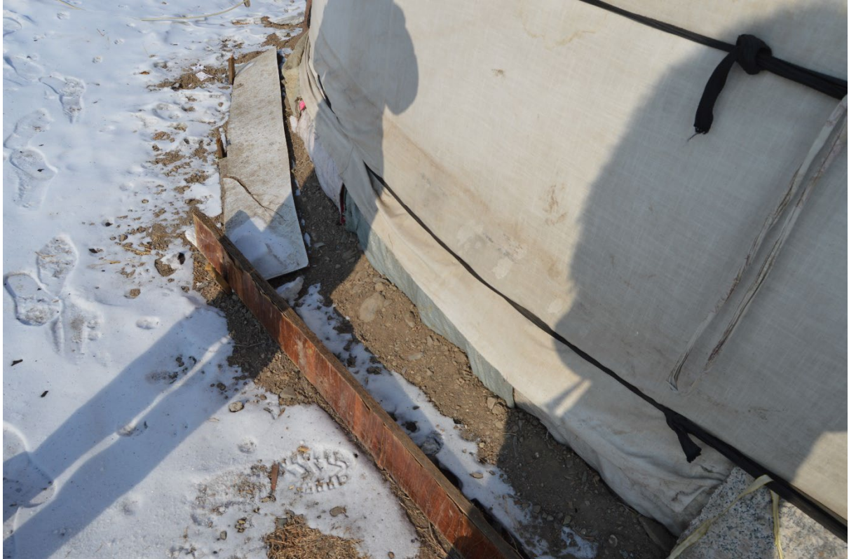
Fig. 2.15 External view of the joint between the wall and the floor of a ger
