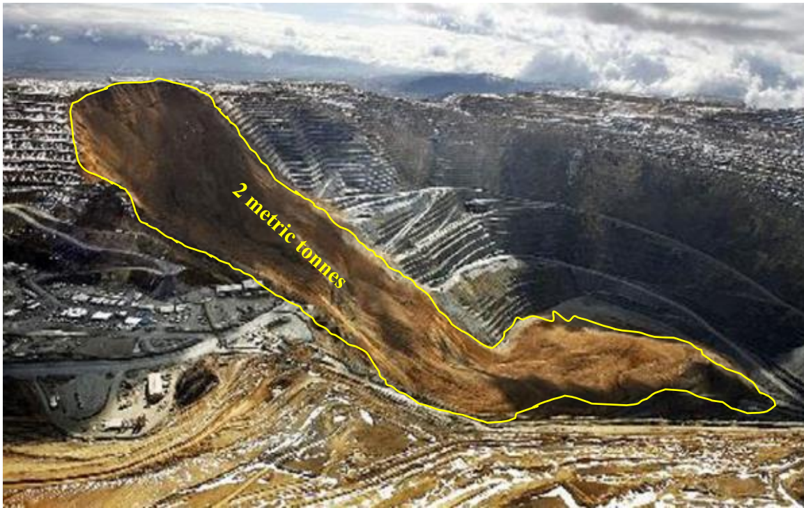
Figure 1.7 A huge failure at Bingham Canyon copper mine in Utah, United States (Parra et al., 2018)
