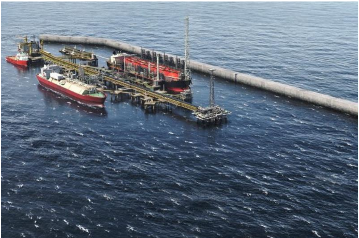
Figure 5-1 Project required 250 piles installations (Courtesy BP)
