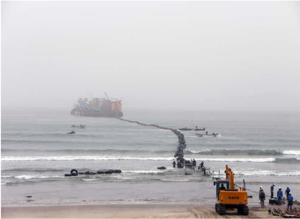
Fig. 1.5 Installation of submarine transmission cables for offshore wind power generation [3]
