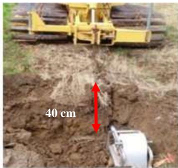
(a) Installing the sheet-pipe in the field
