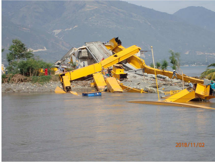
Figure 1.2 The Yellow Ponulele bridge, Palu: (a) Before (September 28, 2018) and after (October 1, 2018) satellite image (modified from BNPB ArcGIS Map service) and (b) Actual picture of the damaged bridge from the site.
