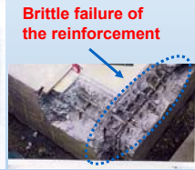
Footing of a Bridge Pier
