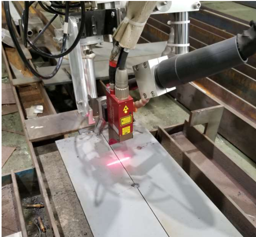
(a) Operating situation
