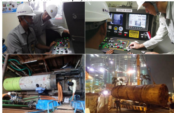
Figure 14. Pipe jacking construction project in Jakarta, Indonesia.
