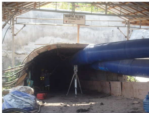
Figure 16. Underground mine portal construction at GDM coal mine, Indonesia.
