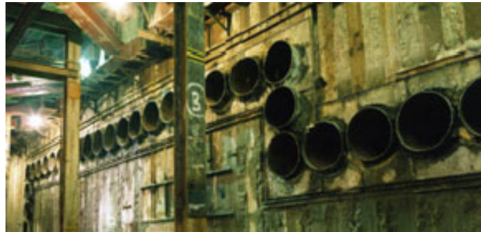
Figure 9. Pipe roof method at tunnel entrance.
