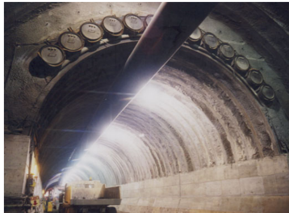
Figure 8. Tunnel entrance with pipe roof method.
