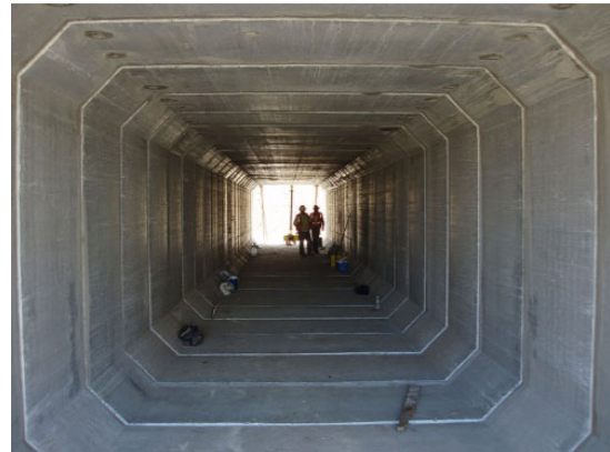
Figure 7. Construction of rectangular pipe jacking.
