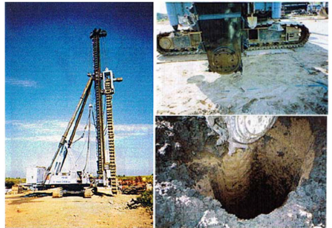
Figure 2. Chain Conveyor Cutter (CCC).
