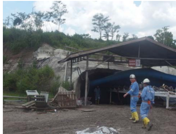
Fig. 3 South Portal of GDM coal mine.
