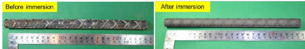
Figure 3.23 A 20-year-old deteriorated reinforcing bar
