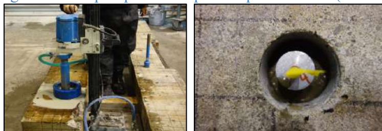
(a) Core drilling
