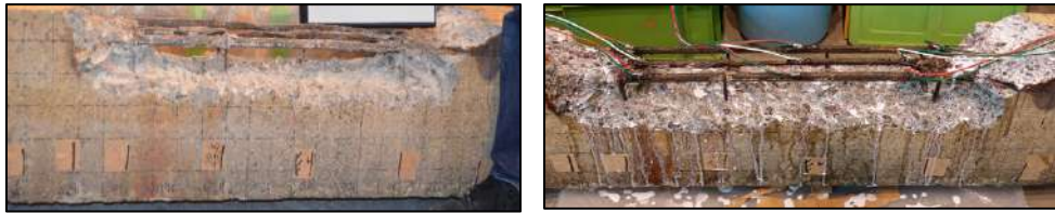
(b) After concrete crushing
