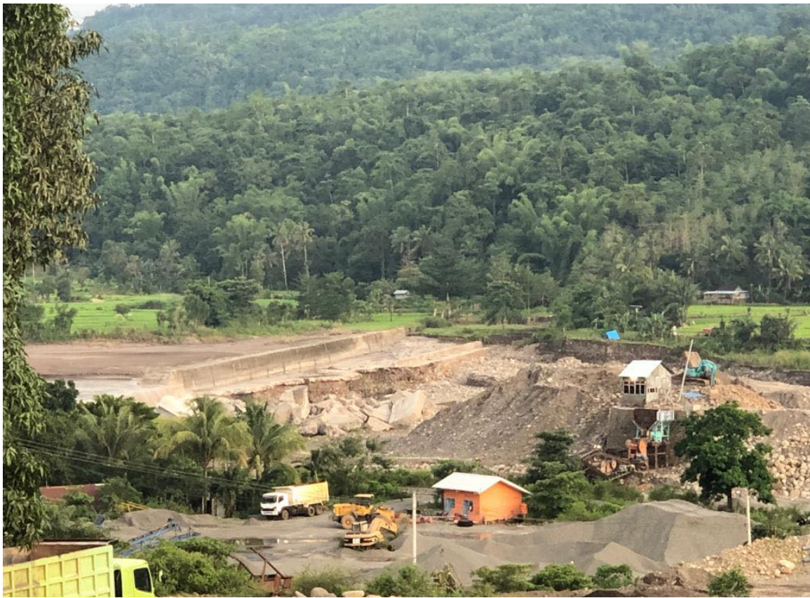
Figure 9 Mining activity caused a damage to sand pocket
