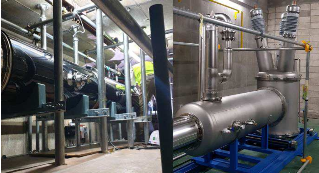
Fig. 1.14 Normal joint box and termination were installed
