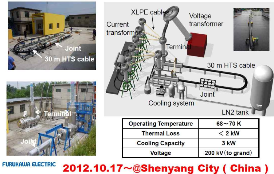
Fig. 1.7 Demonstration of 275 kV/3 kA 30 m-HTS cables in China
