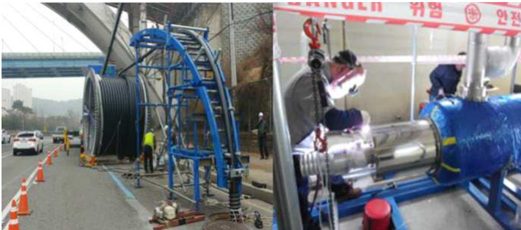
Fig. 1.13 A 23 kV HTS cable installation and joint works at Shingal substation (M/H #1 – M/H #3 section)
