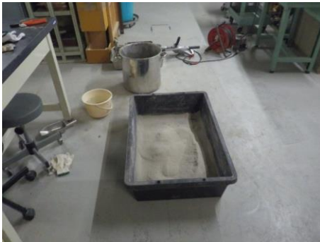
(a) Mix the dry sand and rapid-cement.
