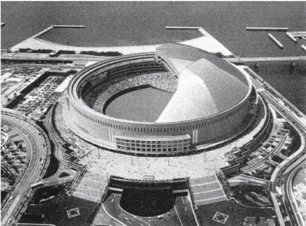
Figure. 1.4. Fukuoka dome (originally named) with a retractable titanium roof [5].
