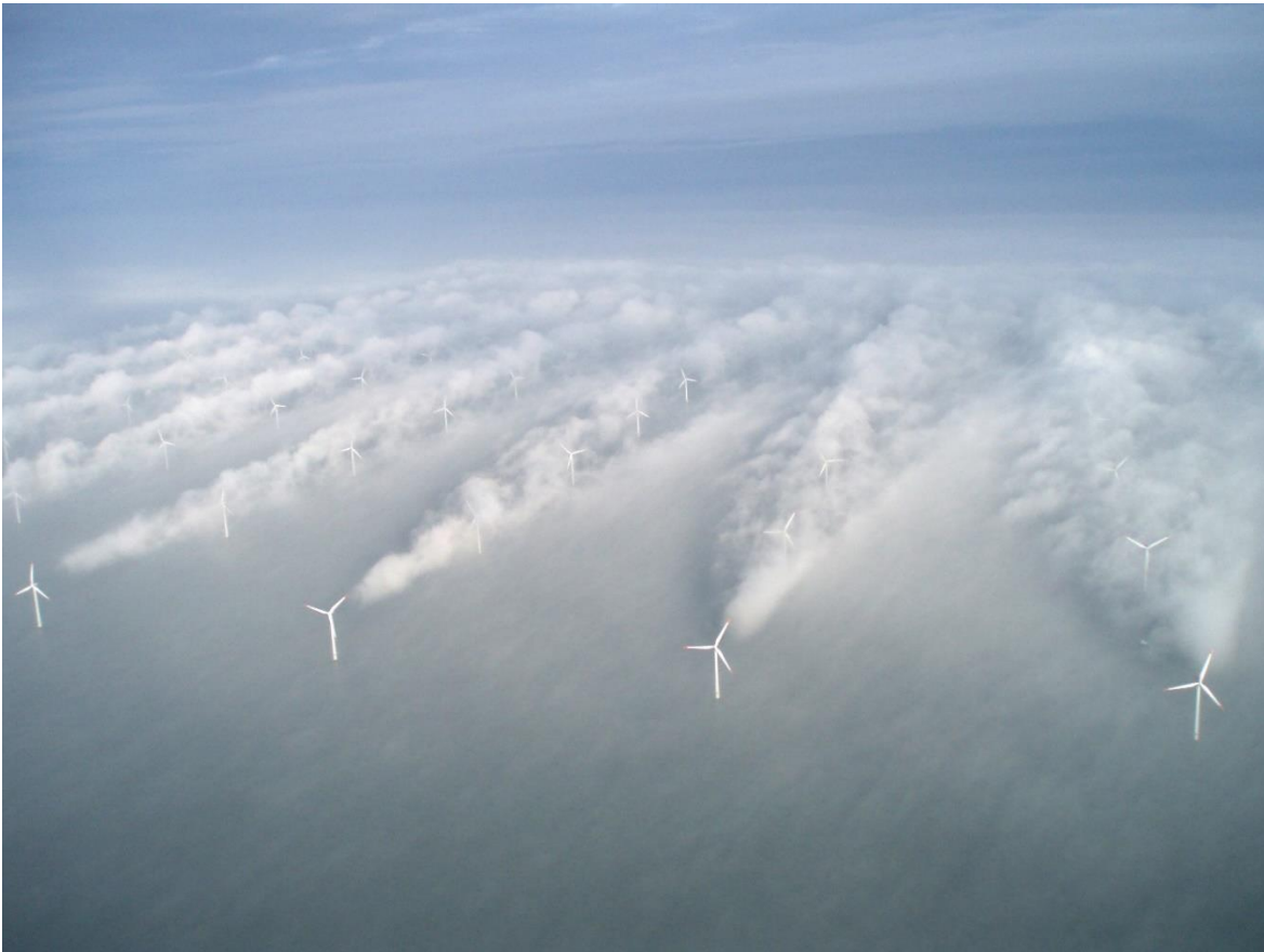
Figure 1.6 Horns rev offshore wind farm [13], where wind-turbine wakes are visible due to fog.
