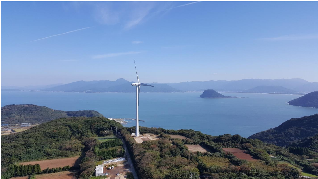
Figure 1.13 Wind turbine in complex terrain.
