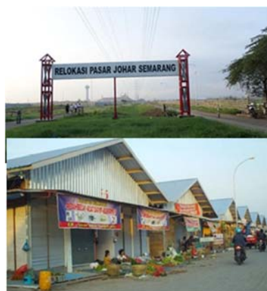
Fig 9: Relocated market, The New Pasar Johar.
