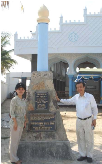
Figure 6 The Firstly Built Tsunami Pole (February 2006) Pole No.: 01, Height: 3.15 m, Distance from Shore: 2.80 km, Location: Gampong Lamdingin, Kecamatan Kuta Alam, Banda Aceh. The placard in front of the pole shows the inundation height, distance from shore, time of tsunami arrival, time of earthquake, location name, words of wisdom, developer, and donor
