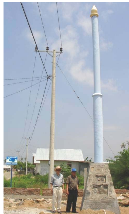
Figure 9 The Tallest Tsunami Pole Pole No.: 69, Height: 9.00 m (w), Distance from Shore: 0.50 km, Location: Masjid Lam Tengoh, Peukan Bada, Banda Aceh. The wave height was justified from witnesses, because there was no inundation mark left by the tsunami.
