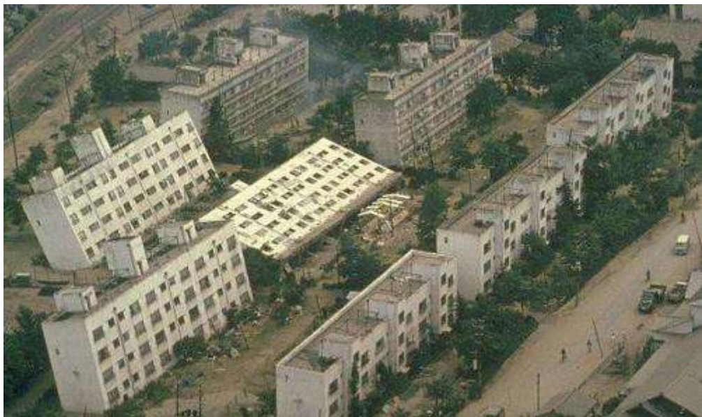
Photo 1.1 Building's collapse caused by ground liquefaction in Niigata earthquake, 1964. (Japan National Committee on Earthquake Engineering)
