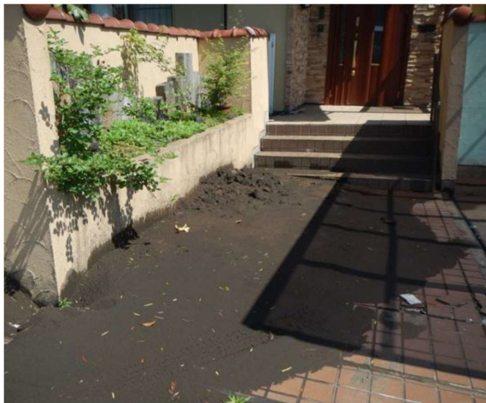
Photo 5.1 The deposition of boiled sand nearby the entrance of residential house (T. Nakano et al. 2017.3)
