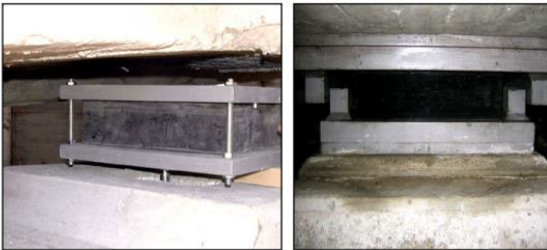
a. Elastomeric bearing with anchor plate
