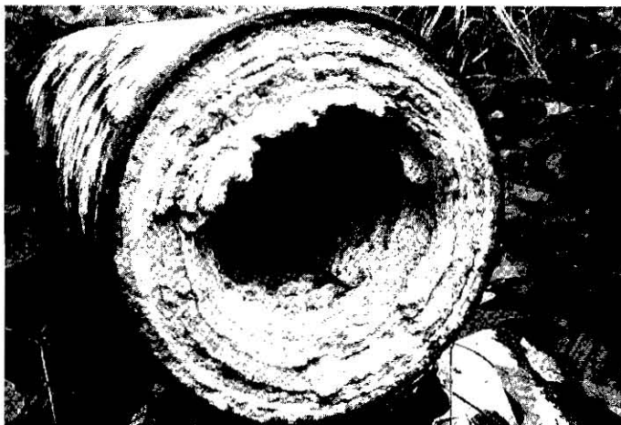
Fig. 1. Occurrence of silica scale deposited on the surface in a pipeline.
