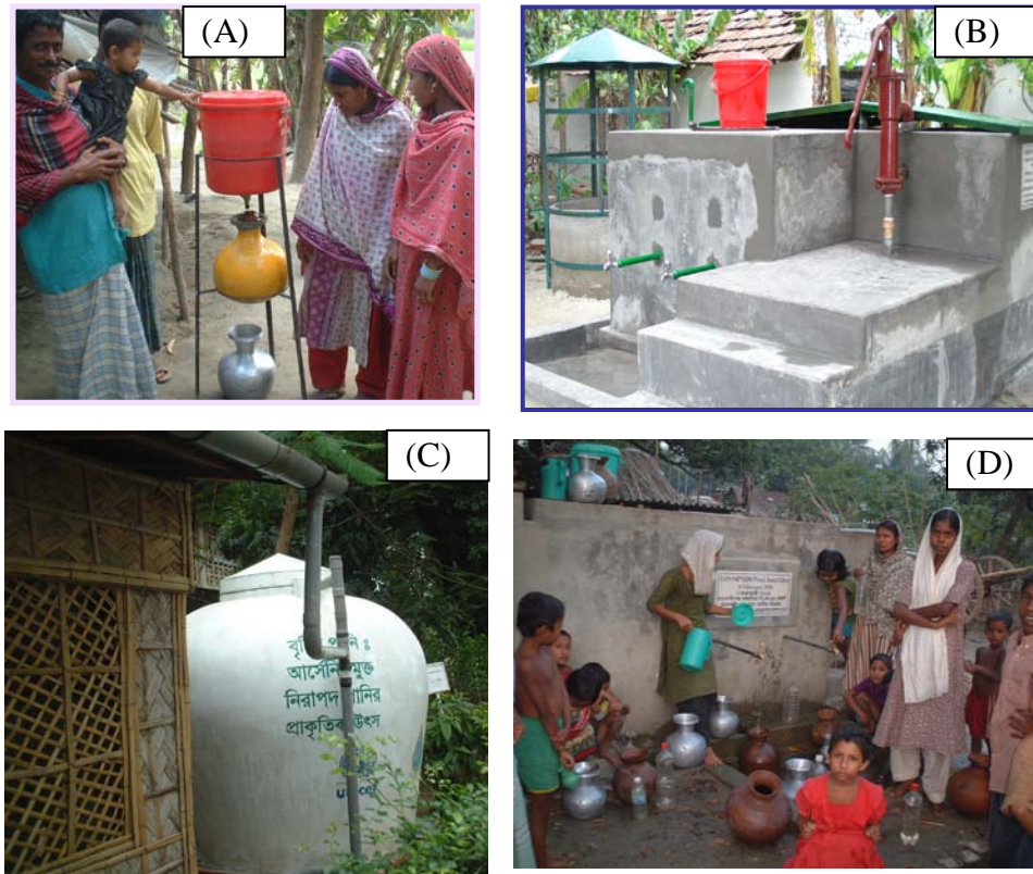
Figure 1.4 Photograph of alternative safe water devices: (A) Household As removal filter, (B) Dug well sand filter, (C) Rain water harvester, and (D) Pond sand filter
